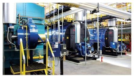
ramingham State University had been carefully planning facility upgrades for over five years. A 1979 Cleaver-Brooks water tube boiler (1,000 HP) was producing steam to the campus with an original burner that was only capable of burning #6 fuel oil. Achieving significant energy efficiency, maximum cost savings, and reducing emissions was of critical importance and considered long overdue.
